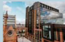
2 The Main Site Tower
